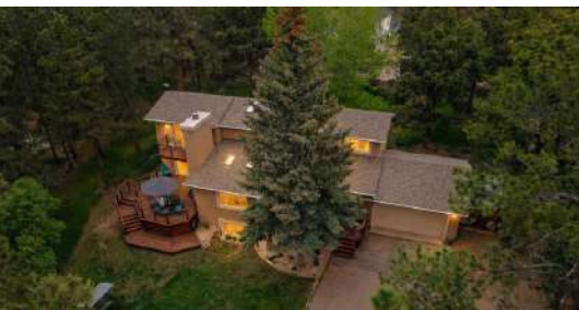
1540 Fawnwood Road Monument, CO 80132
