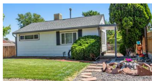
1570 Shoshone Street Denver CO 80223
